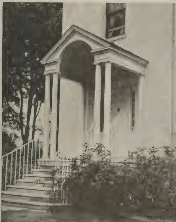
DETAIL OF ENTRANCE AFTER ALTERATIONS.
